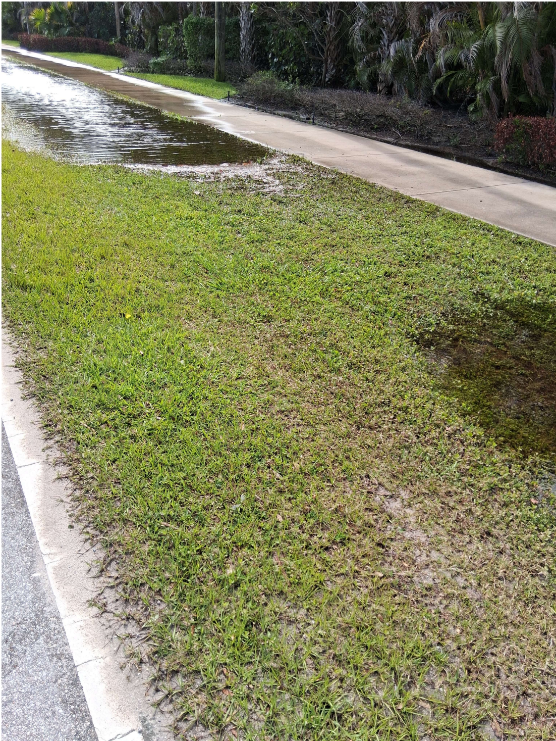
Old Winter Beach Road swales post-heavy rain events over multiple days.
